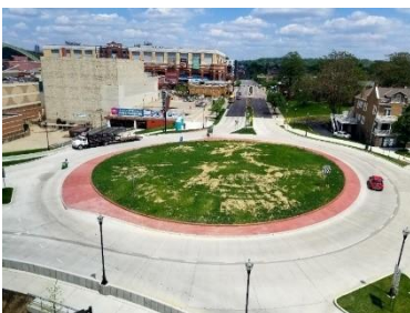
Newport, KY Roundabouts
